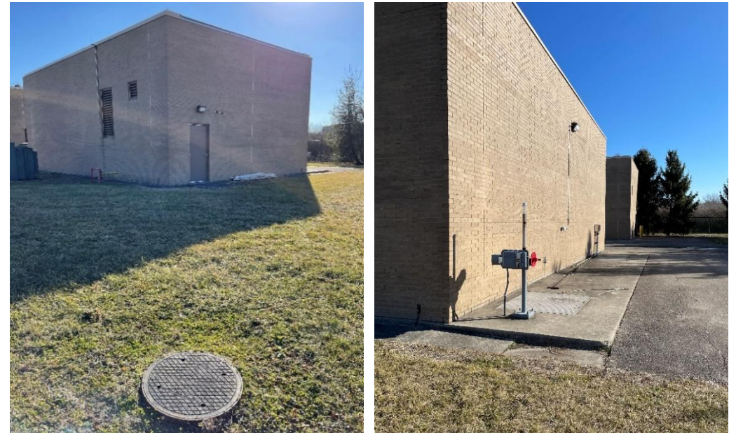
Page Manor Lift Station
