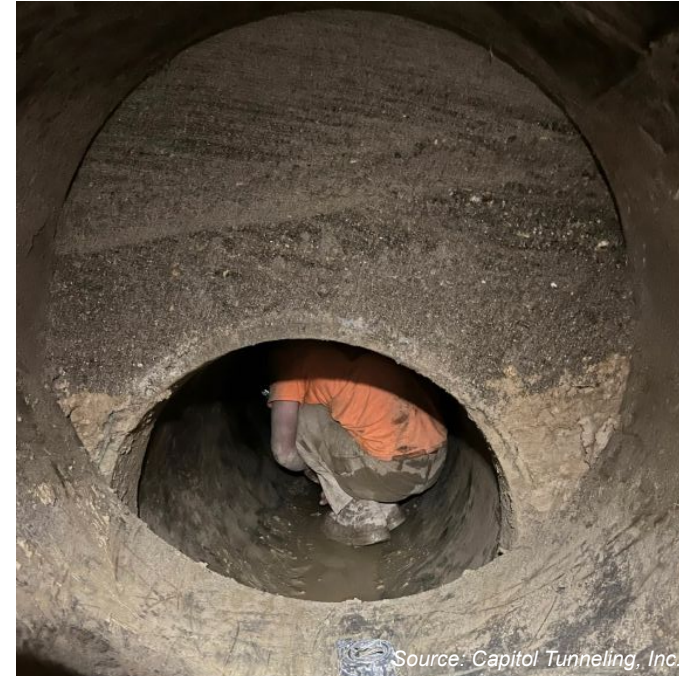
36" Steel Casing From the West
