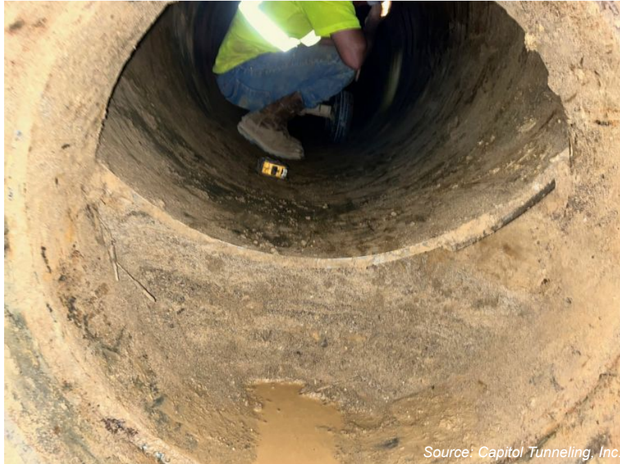
30" Steel Casing From the East
